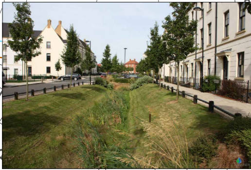
Insets between the North and South parcels of the site can be used to drain excess flow, whilst utilising the green band beneath the overhead cables
