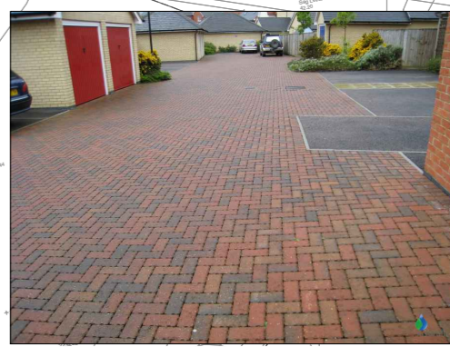
Porous Paving to be used for all private driveways to provide water quality treatment in accordance with CIRIA Guidelines
